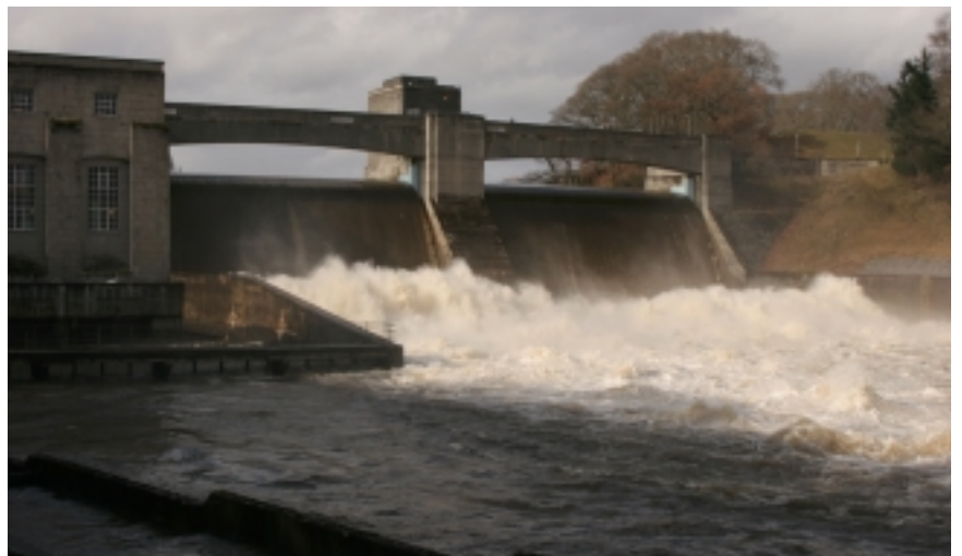
The hydro electric power station at Pitlochry operated by Scottish & Southern Energy plc
