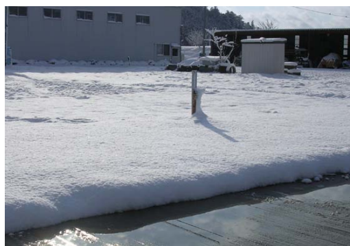
The ICAX technology has been licensed by Misawa in Japan for this experimental site at Hiroshima, where the area to the front of the picture is being kept free from ice and snow using heat captured during the Summer.
